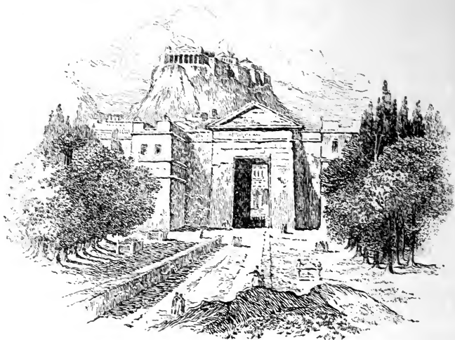
WALLS OF ATHENS — RESTORED
